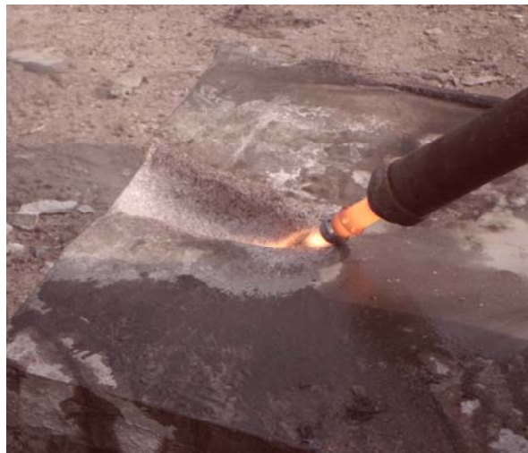
Figure 4 – Formation of slotted working by using BVR60 Thermal cutter torch with gas-dynamic nozzle
