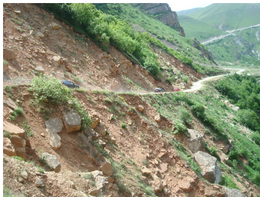
Figure 8 – The road to the Khinalig village
